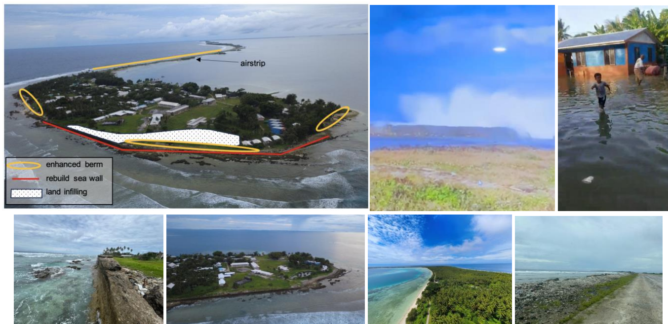
(top row L to R): Overview of available options for coastal protection at Jabor, Jaluit Atoll, overtopping of the seawall during a high wave event and subsequent flooding in the village. (bottom row, L to R): The ageing WW2 era seawall, Jabor from above, the north coast of Jaluit, Jaluit and the vital, yet highly vulnerable airstrip.
